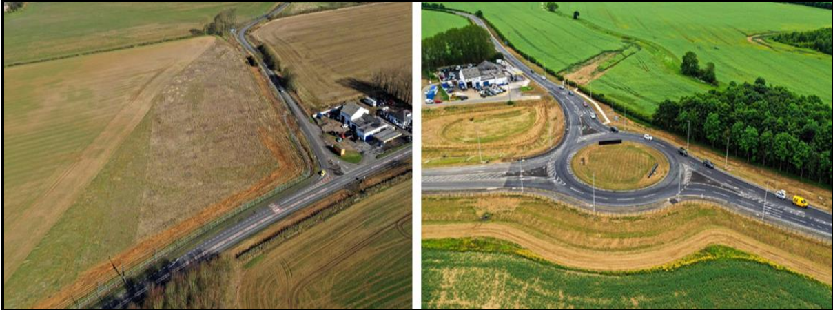
A46 Dunholme/Welton Roundabout – Before and After
