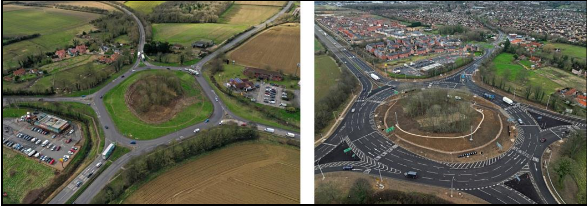
Holdingham Roundabout – Before and After
